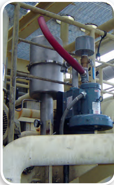
Shin Nippon Steam Turbine Stainless Steel Vacuum Assisted Oil Mist Eliminator
